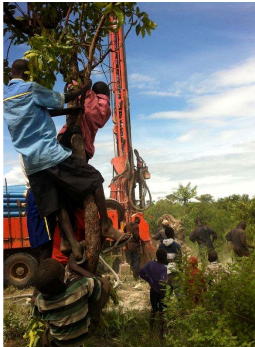
Note boys in tree watching drilling.
